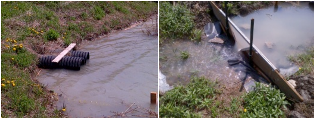
Figure 6 - Site 2 pond outlet and constructed weir during an overflow event
