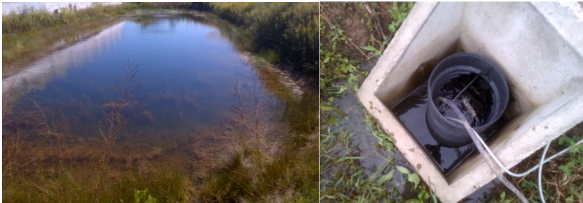
Figure 7 - Site 3 pond and overflow outlet showing sample intake tubing for autosampler
